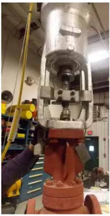
Hydraulic actuator attached to a process valve.
